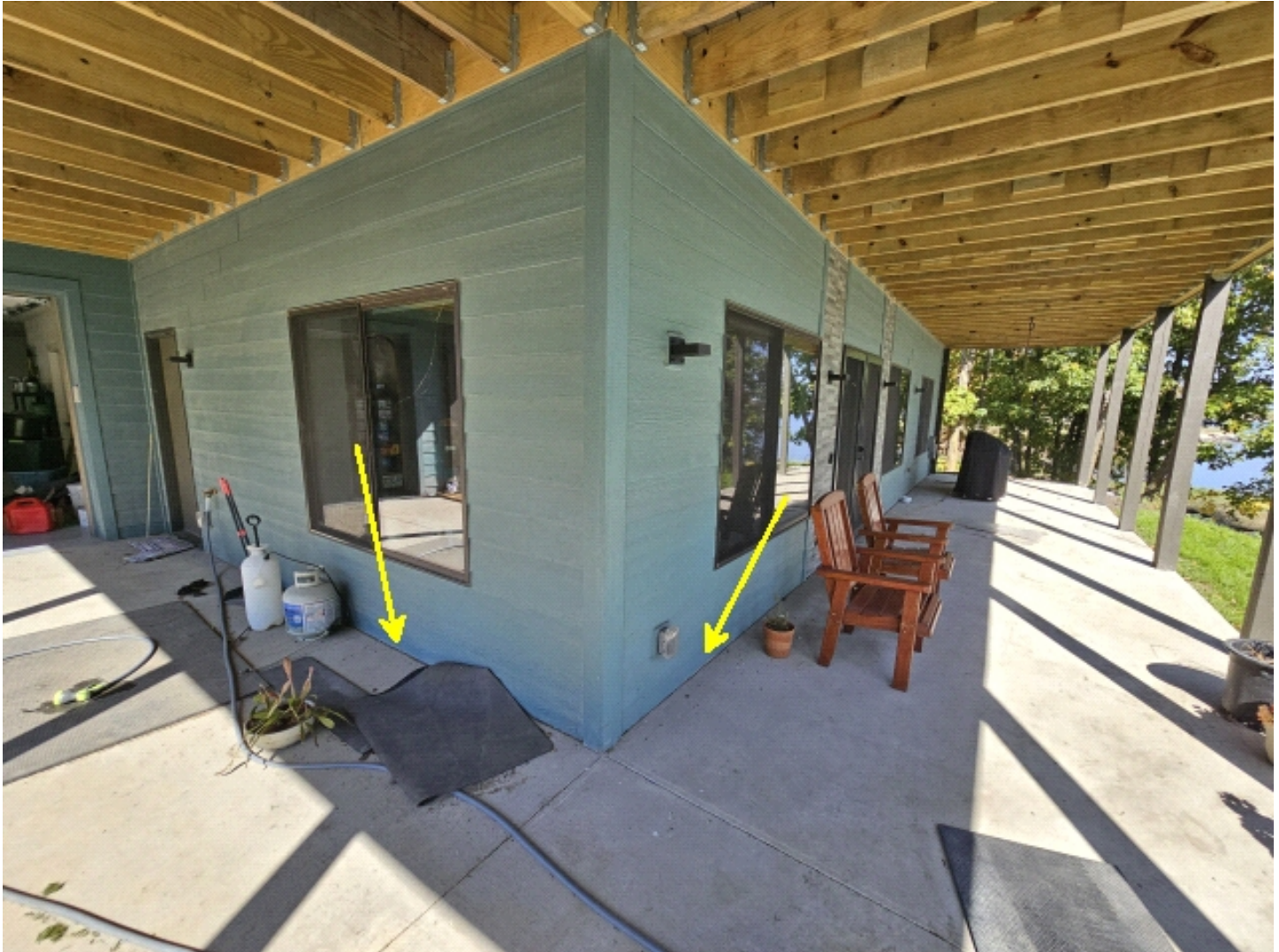
1" Clearance from concrete is specified by LP SmartSide.
