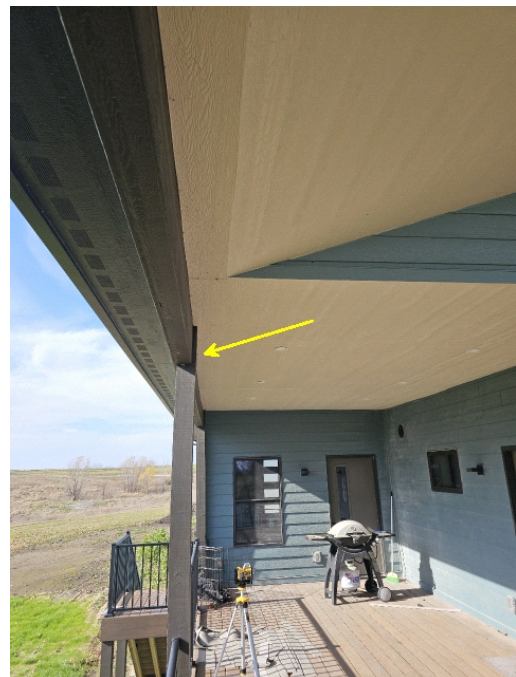
Beam bows out approx 2" in the center of the span.
