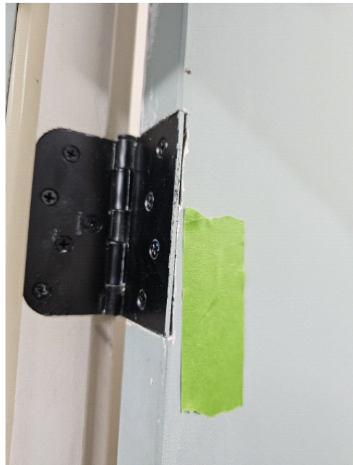
Builder hacked out hinge pockets in an attempt to make adjustments to a door that is not correctly set plumb, level, and square.
