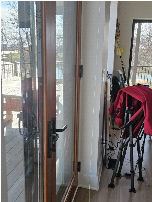
Deck door out of plumb.
