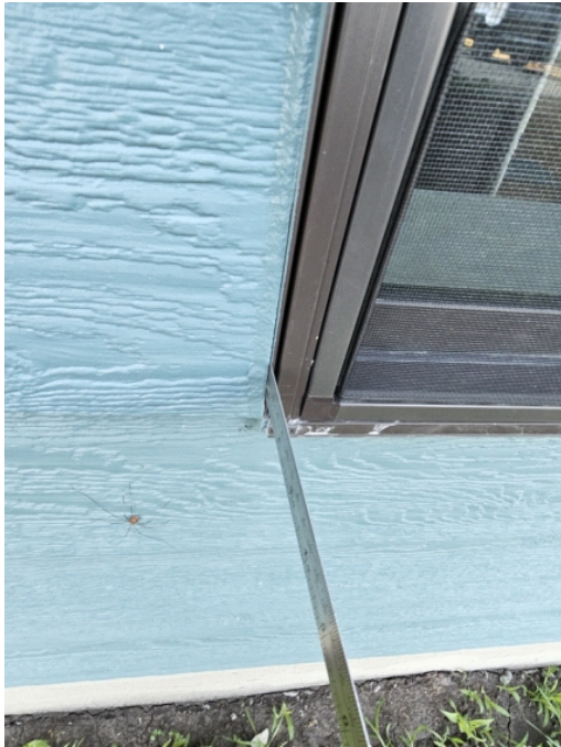
Required 3/16" gap was not left at the window
