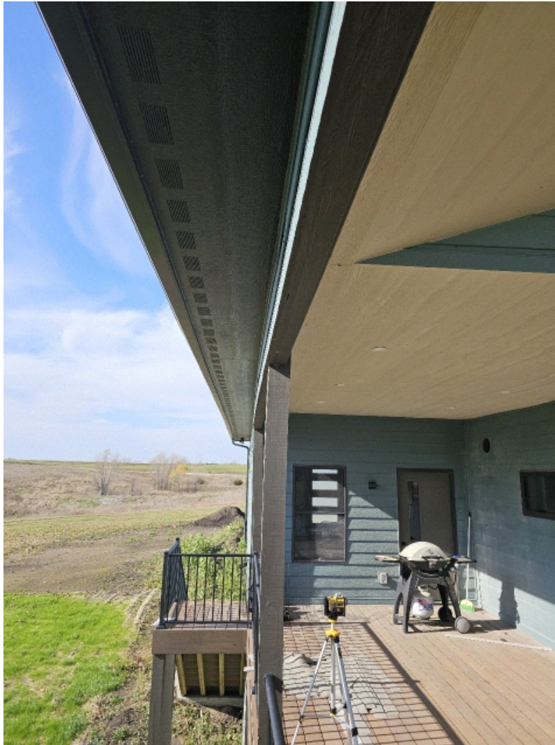
Beam has notable bow outward at center of span.
