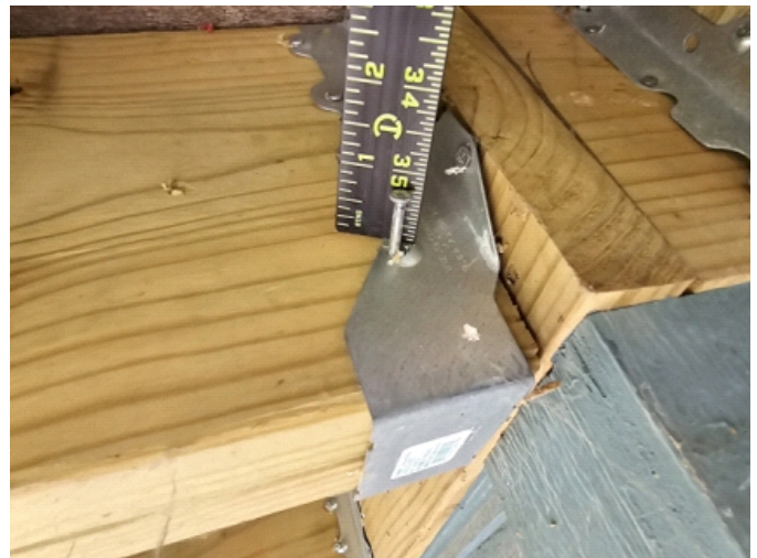
1.5" nails used at angle holes
