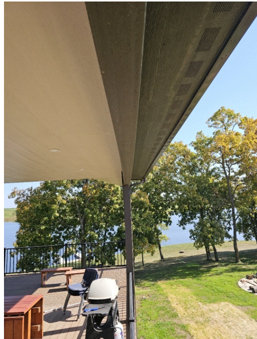
Beam bows outward at bottom over span. Beam rotates outward at bottom towards center.
