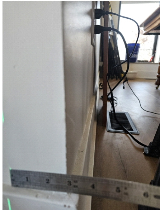
Back wall is out of plumb, approximately two and three quarter inches from top to bottom.
