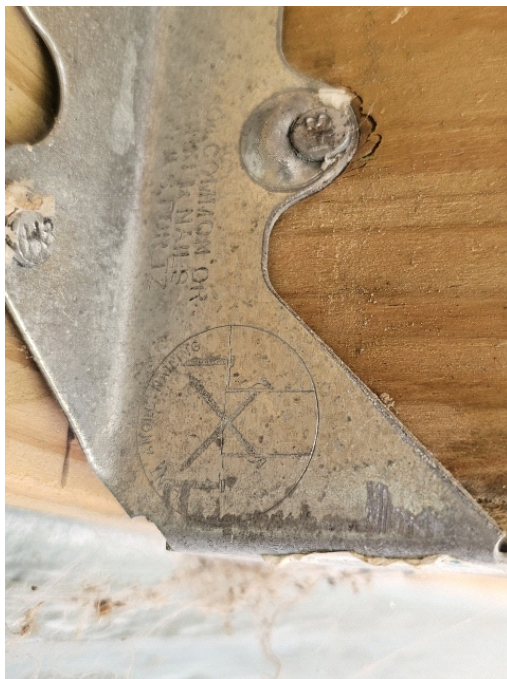
Joist hanger shows longer nails to be used at the angle holes. The builder ignored this instruction.
