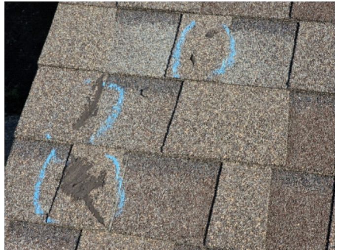
Replace damaged shingles.
