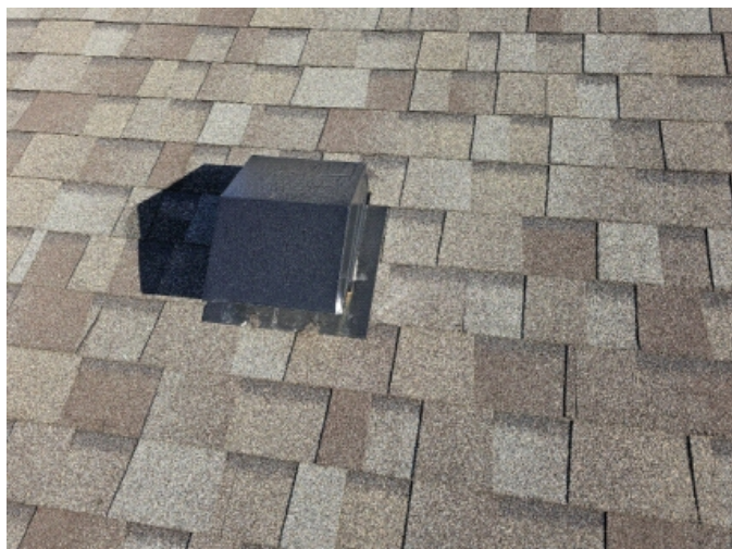
Vent hood not installed into shingles correctly.
