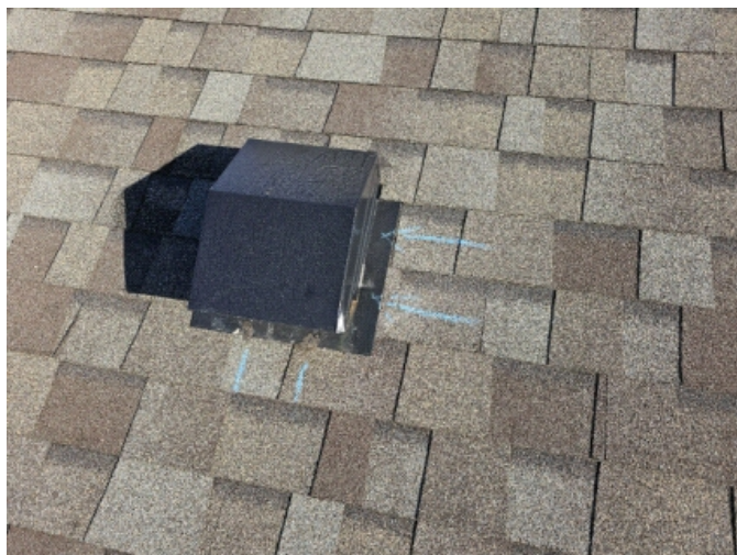
Shingles should lap onto hood at blue arrows. Hood should be nailed to the roof under shingles. Nails at bottom should not be there.
