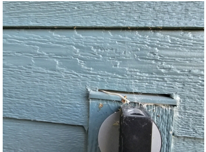
Wire inserted into the non-sealed joint.
