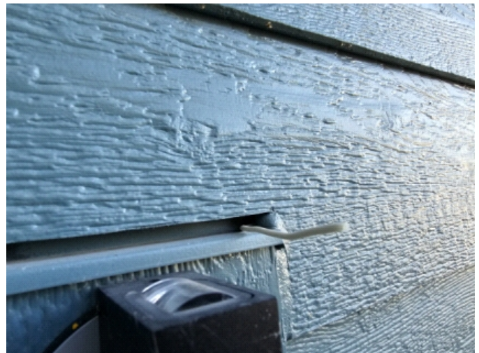
Wire inserted into the non-sealed joint.
