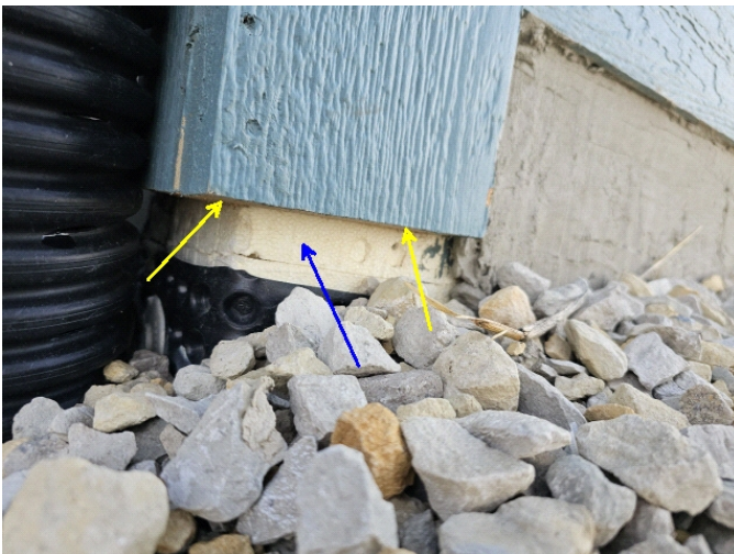
Exposed ICF, blue arrow. LP SmartSide trim edge left exposed, not properly sealed and painted at the cut edge, which is a requirement of LP SmartSide, yellow arrow.
