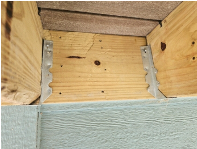
Deck rim joist is attached with 3 nails at 16"o.c. This deck connection to the ICF's is deficient
