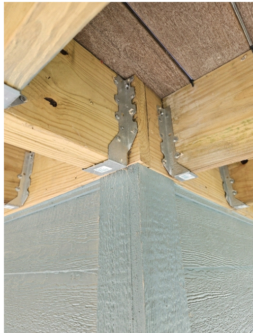
Beam bearing hanger installed too close to end of supporting member. Nails are splitting wood , attachment is in question.
