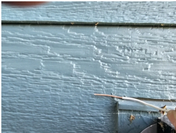
Wire easily inserted behind the siding, this is an open path for moisture to intrude behind the face of the siding.
