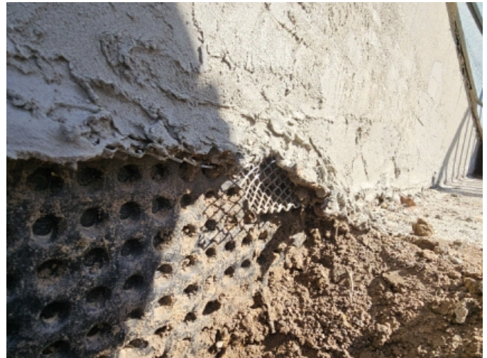
All metal lath is to be fully encapsulated in scratch coat to protect against exposure to the weather.
