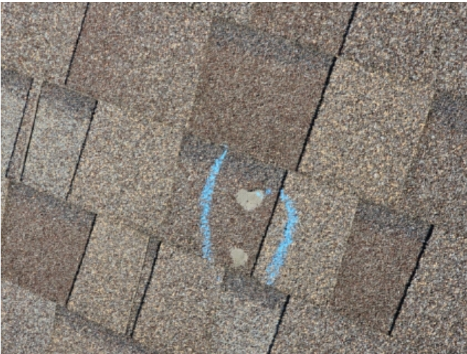
Replace damaged shingles.
