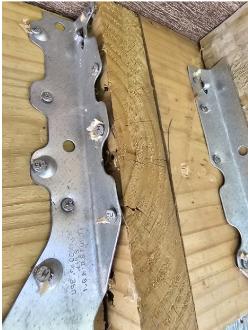
Wood is splitting at nail. Nails used are too short.
