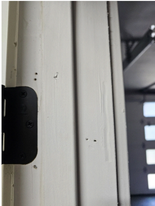
Nail holes in trim are not filled.
