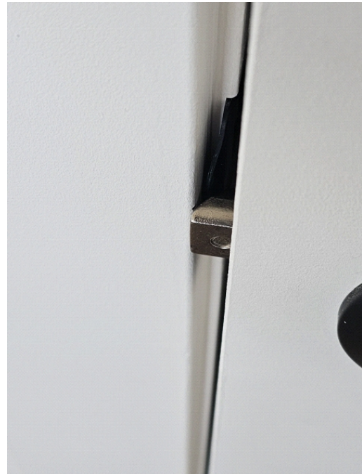
Doors should have extended strike plates. Latch drags on finished wall and scores and damages the surface.
