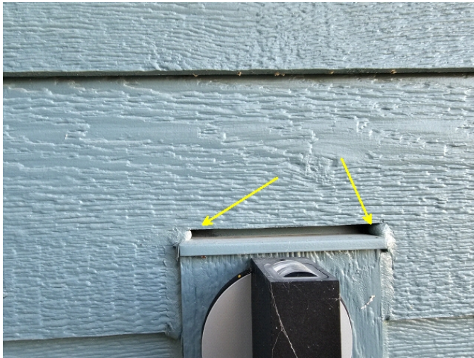
End dam sealant not complete at the edges of the metal flashing. This is a moisture pathway behind the siding Which could lead to moisture intrusion into the ICF wall.
