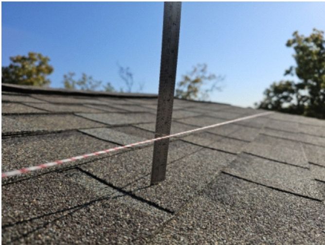
2.5" dip in roof measured.
