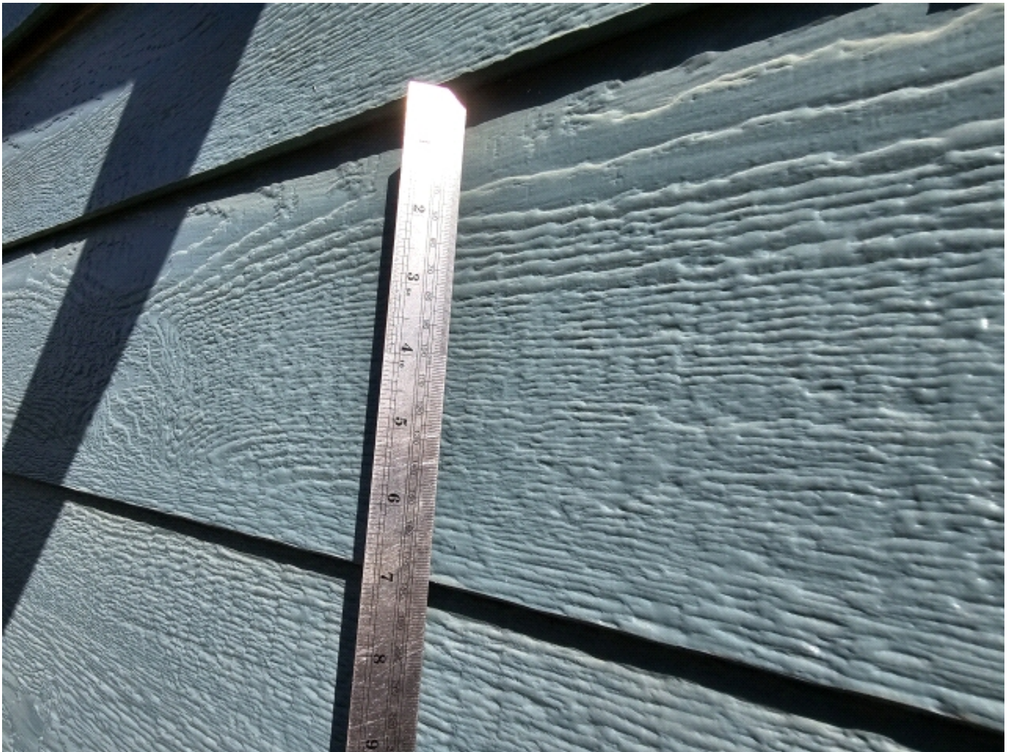
Siding is LP SmartSide 8" horizontal lap siding.
