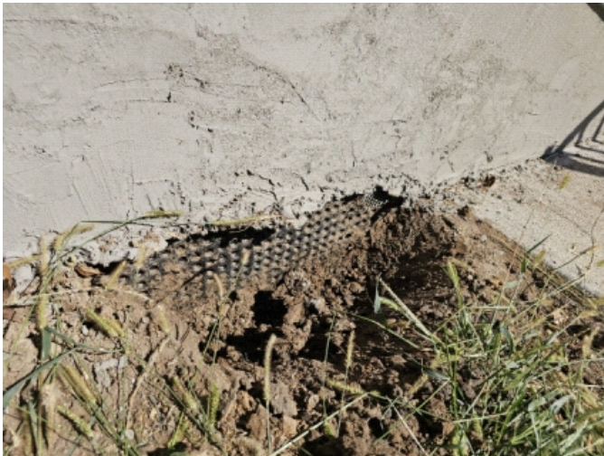
Wire lath exposed, not terminated correctly at base.
