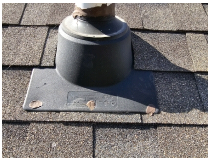
Shingles should lap onto hood at blue arrows. Hood should be nailed to the roof under shingles. Nails at bottom should not be there.
