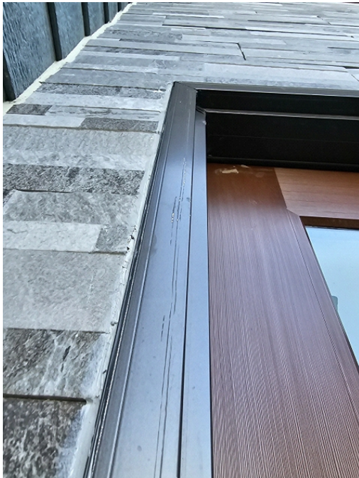
Looks like the door was drug across the ground damaging the finish and leaving grooves in the metal.
