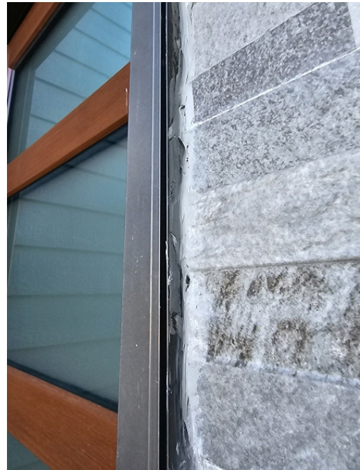
Sealant smeared on door frame.
