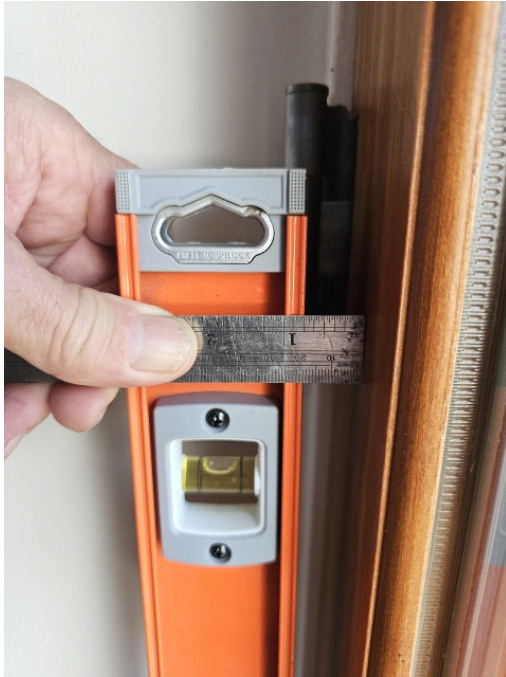
Deck door out of plumb.
