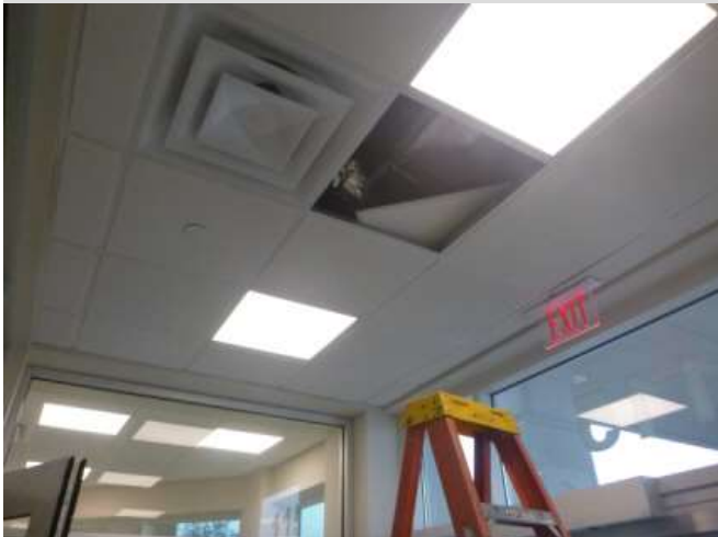
Removal of tile to inspect leak area.
