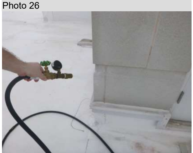
Water test of stone joints
