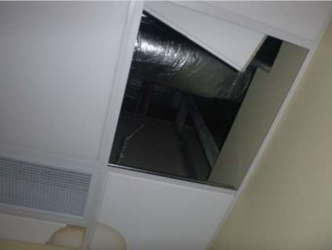
Tile removed for observation during testing
