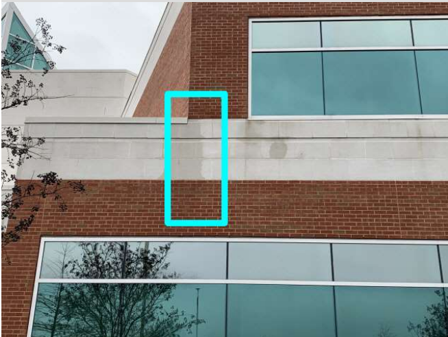
Roof to wall transition
