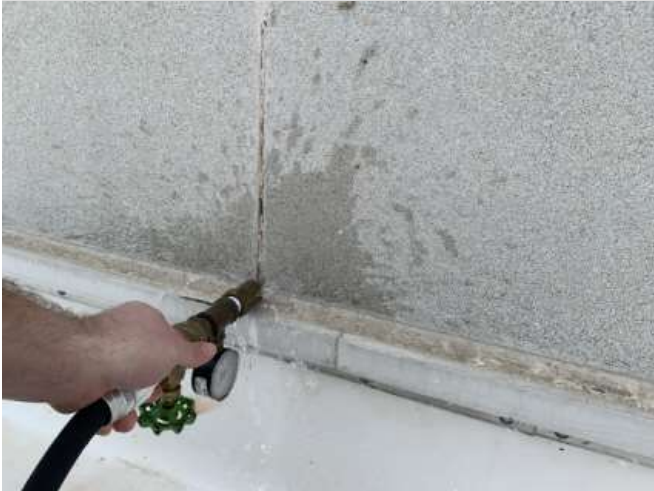
Water test in progress
