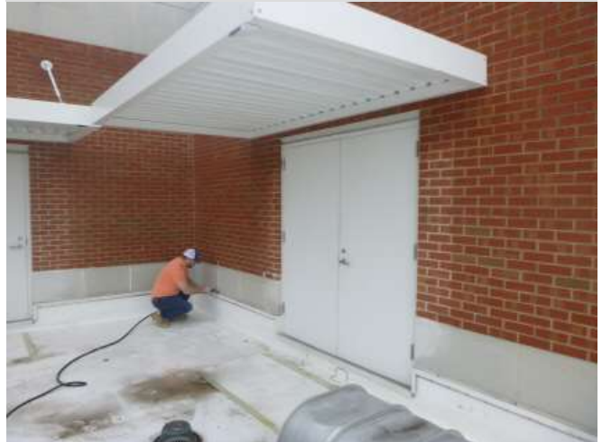
Water test in progress
