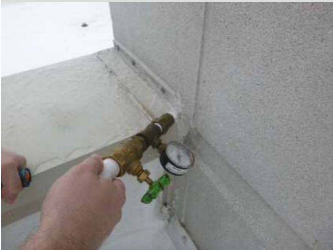
Tests of flashing terminations did not produce visible leakage
