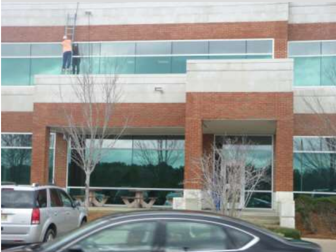
Water test area
