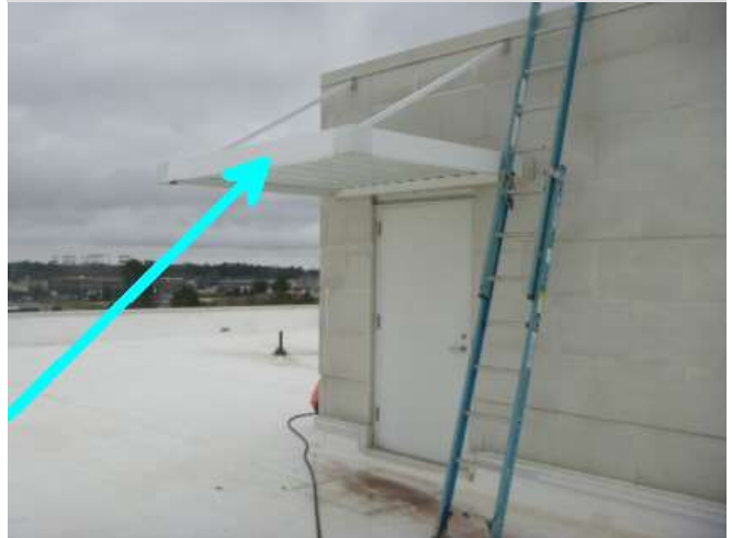
Awning has been installed to reduce door exposure to weather.
